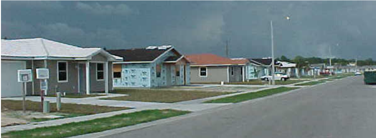
Street scene showing the three closest homes (from left: white "barrel" s-tile (RWB), terra cotta s-tile (RTB) and white metal (RWM)).
